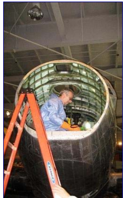
1005hrs: Steve Bravo puts on the first spray of anti-corrosion material
